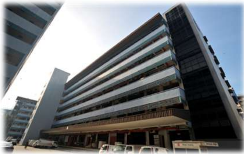
Toa Payoh North 1 Cluster before redevelopment
