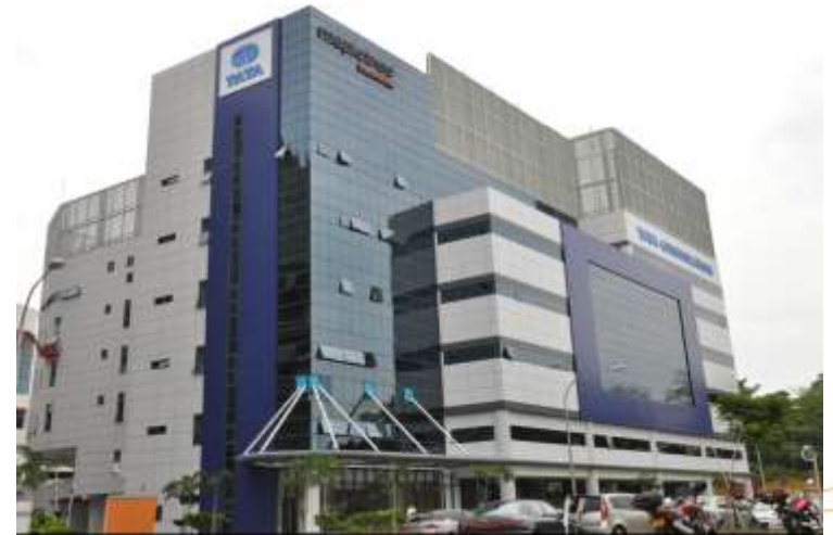
Example of BTS – Tata Communications Exchange
